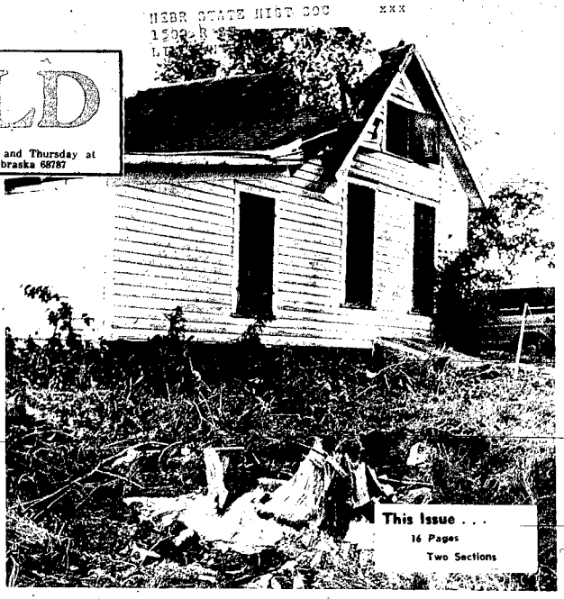
VIVID EVIDENCE of the strength of the storm is this farm home of Chuck Victor five miles south and one-half west of Concord. The storm toppled a large tree onto the house, causing considerable damage.
